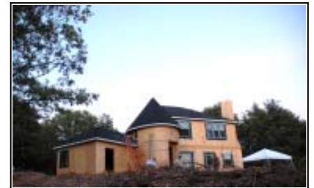
My new residence, under construction summer, 2006
